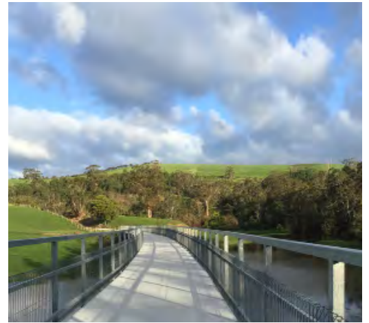
Rebuilt surface on historic timber trestle bridge over the Tarwin River.
