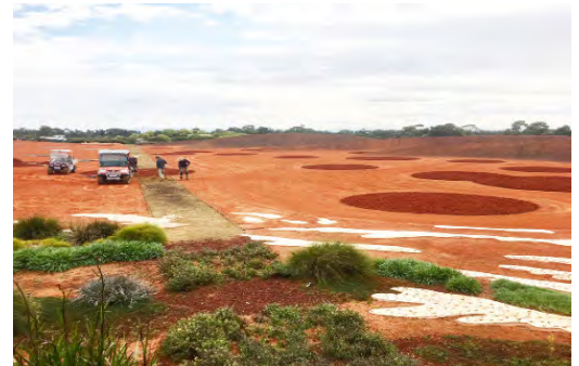
New growing media, edging and mulch ready for planting in autumn 2019.
