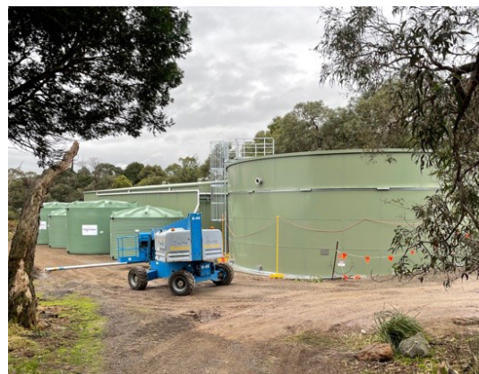
Our new recycled water treatment plant and 500kL storage tank will take us off potable water for irrigation Photo: Chris Russell
